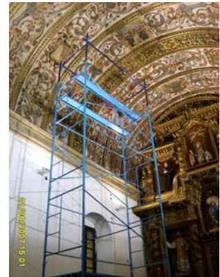
Fig. 8. View of the ceiling of the chapel
