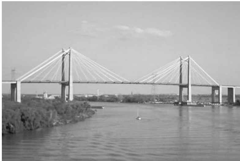
Fig. 3. View of the Zárate Bridge in Argentina
